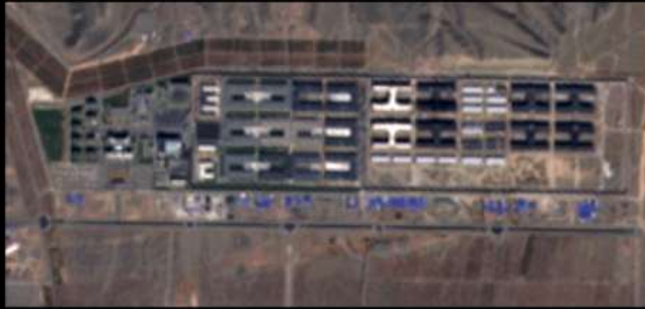
This image, taken by Sentinel Images in October 2018, shows how quickly the site has been developed
